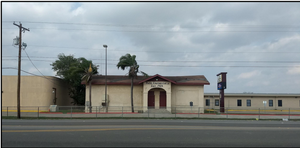
Figure 1: Old Main Entrance to Runn Elementary School in Donna, TX
